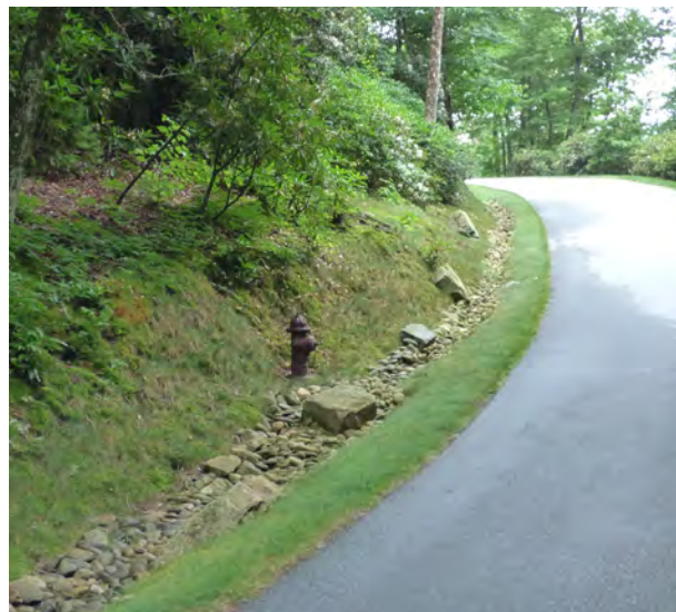
Example of a rock lined swale with check dams designed to slow the flow of stormwater
